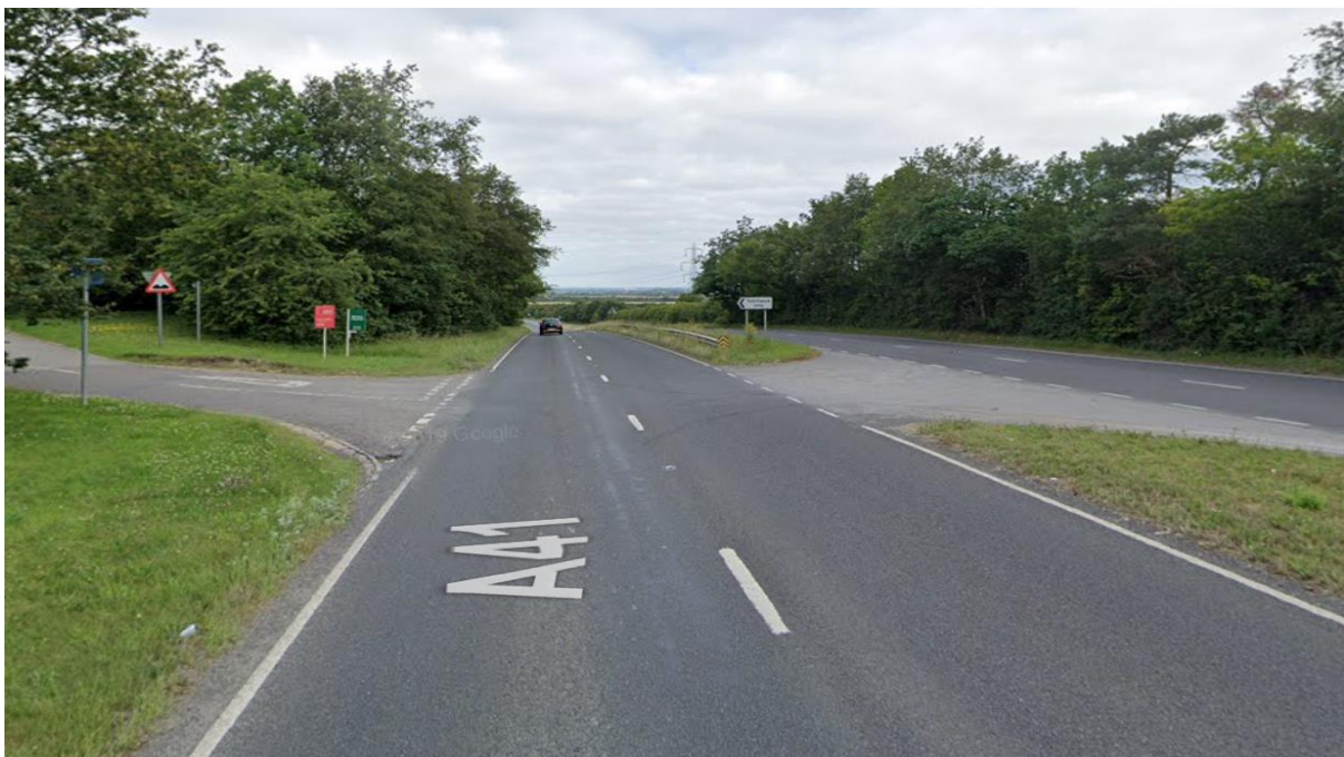
Westbound approach – No U-Turn on central reserve
